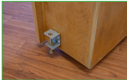
Outswing, support bolt bracket
